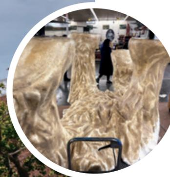
**FEBRUARY 2023:** The bottom of the mammoth is pictured after an initial coating. Once the structure was carved from foam and supported with steel, artists covered it with layers of fiberglass and epoxy resin and used primer, automotive paint, and a clear coat to create the mammoth's color. (Photo courtesy of Taylor Studios)
